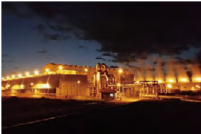
Geothermal Power Plant
